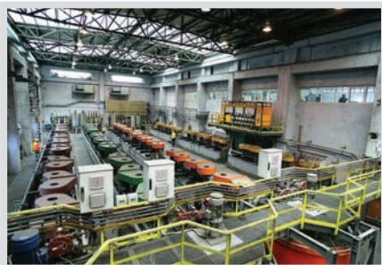
Olympias Processing Plant
