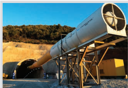
Main Access Portal at Olympias
