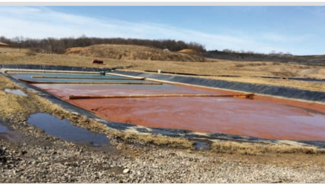
Metal rich sludge settling out in cells allowing clean water discharge at far end.
